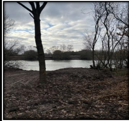
Another view of Upshers showing one of the 16 swims under construction.
